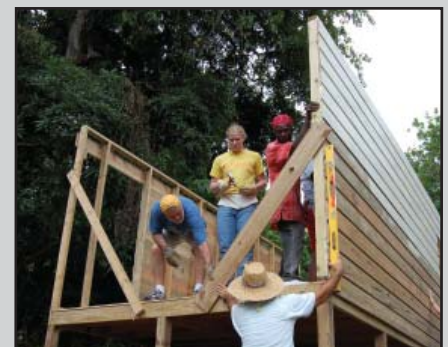
Members of the Jamaica team construct a house.
