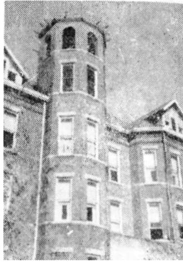
This is a front view of the tower as it is now.
