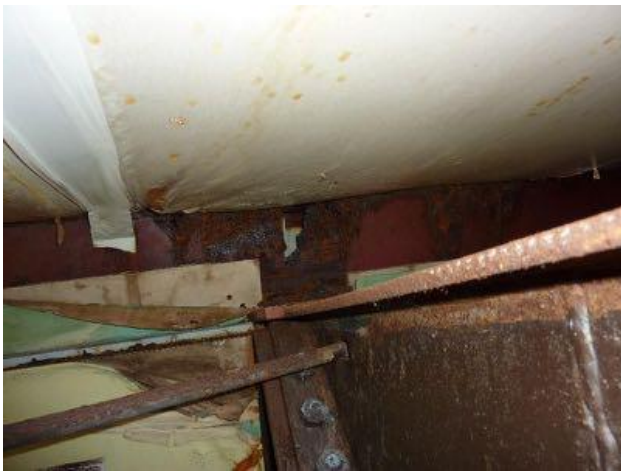
Corroded Steel Roof Purlin (beyond)
