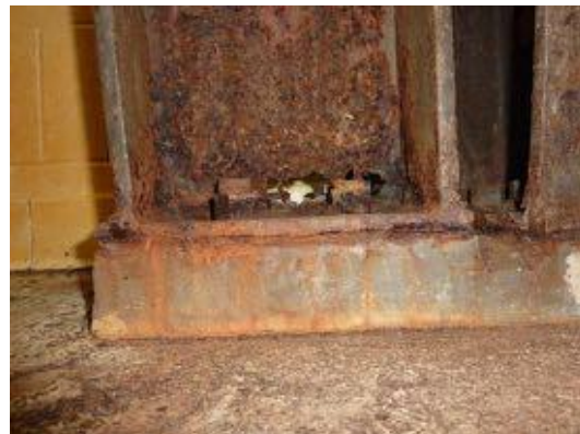
Corroded Flat Portal Frame Column Base
