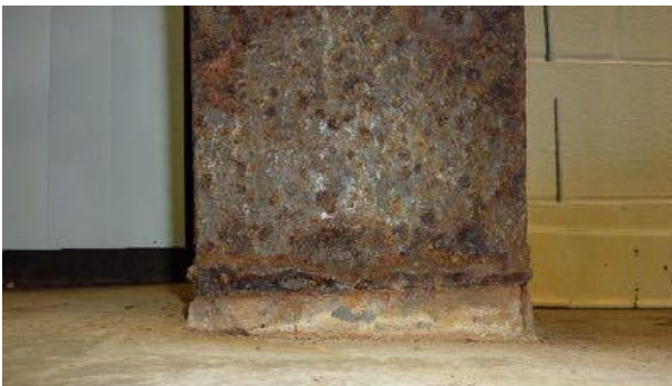
Corroded Gabled Portal Frame Column Base
