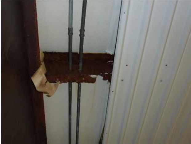
Corroded Steel Roof Purlin
