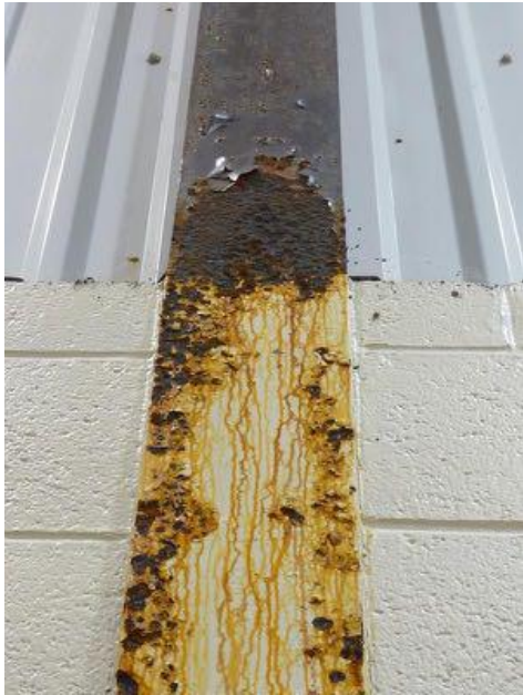
Corroded North Load Bearing Wide Flanged Wind Column
