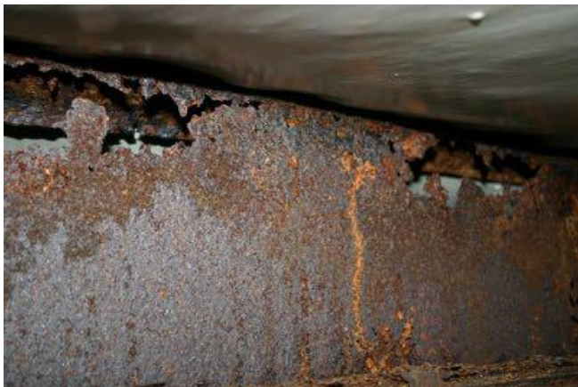
Corroded Steel Roof Purlin
