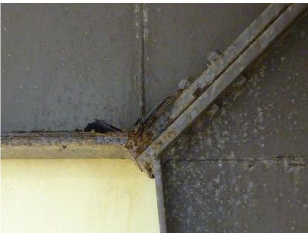
Corroded Flat Portal Frame Girder (west col line)
