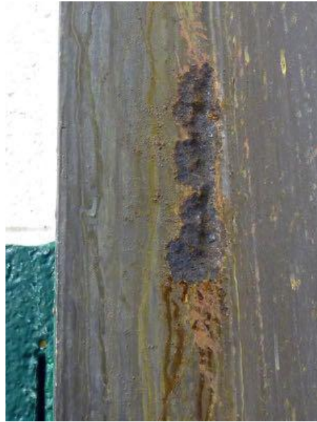
Corroded Gabled Portal Frame Column
