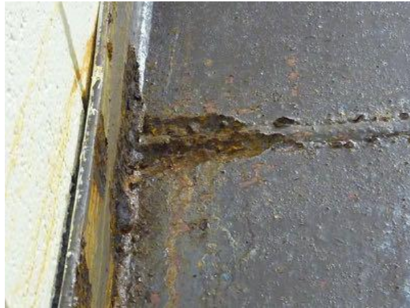
Corroded Gabled Portal Frame Column
