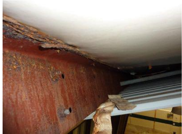
Corroded Steel Roof Purlin
