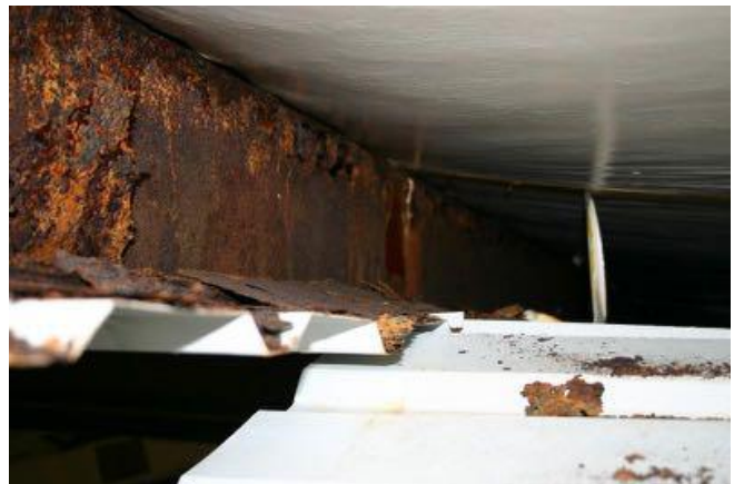
Corroded Steel Roof Purlin
