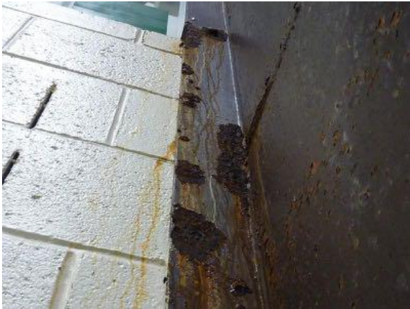
Corroded Gabled Portal Frame Column
